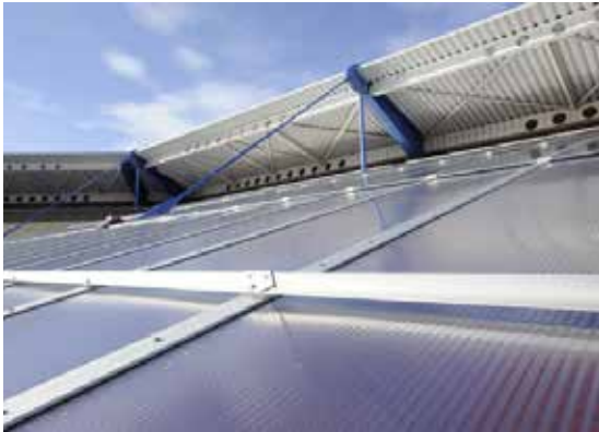
The ink-jet marks the UV-protected side of the sheet.
